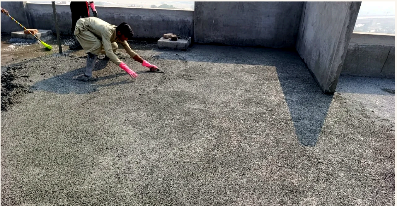
Roof screed application from the SEED Chemicals site archive.
