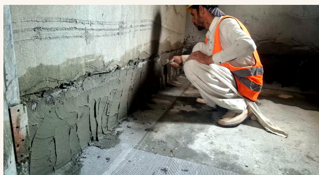
Mesh and coating at a wall-to-floor junction.
